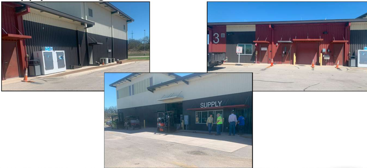
West Side Operation Center Supply Building Drainage Improvements (IFB)
